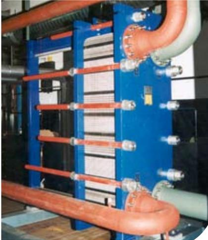
SWPHE as an evaporator in a brewery installation.
