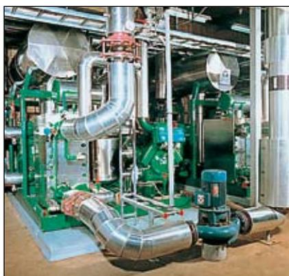
The AlfaRex TM10-B ammonia evaporator and condenser in a chiller heat pump system with ammonia as refrigerant installed in a Danish research institute. The system was built by Sabroe.
